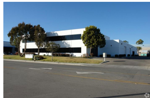
Industrial property. Source: LoopNet
