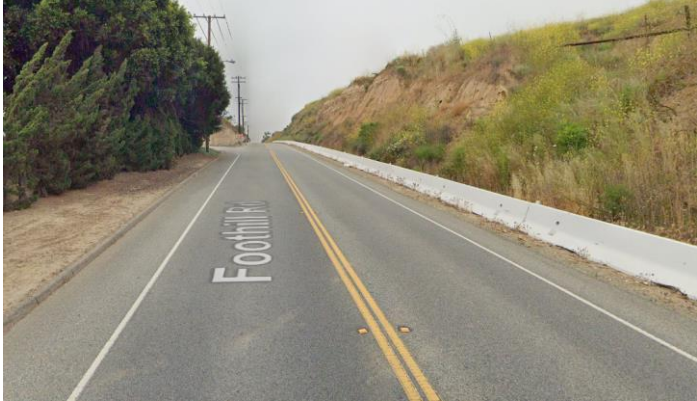
Very Inadequate PES, Foothill Rd
