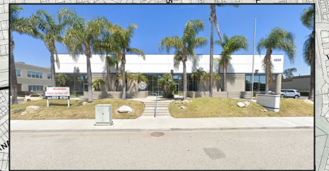
Light Industrial/Flex Change from General/Heavy Industrial and Commercial
