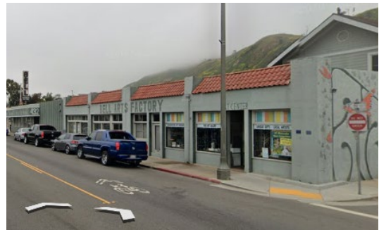
Consistent street wall with minimal setbacks. Source: Google Maps
