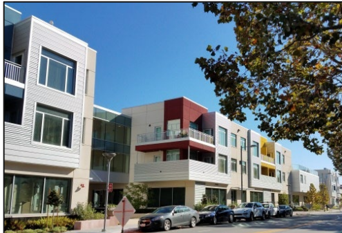
T4.10 (Urban General: West Saticoy) Up to 3-story mixed-use and higher density residential infill development
