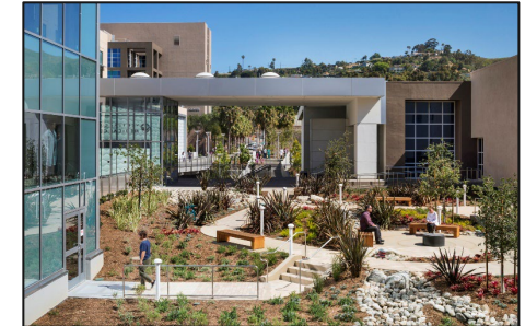
H: Hospital Up to 3-story medical care and adjacent services/uses
